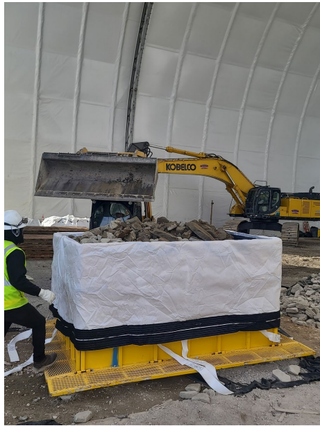
9 CYD Bag (20,000 lb.) Bag in Custom Lift/Loading Frame
