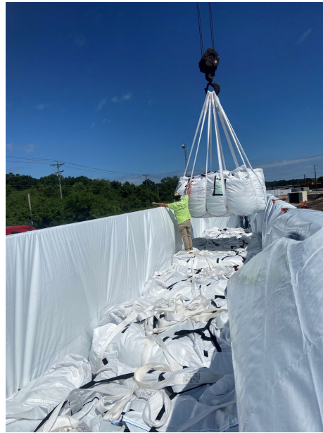
9 CYD (20,000 lb.) Bag Commercial Nuclear Power Plant Remediation Project
