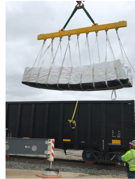
25 CYD (50,000 lb.) Bag North-East Nuclear Decommissioning Project
