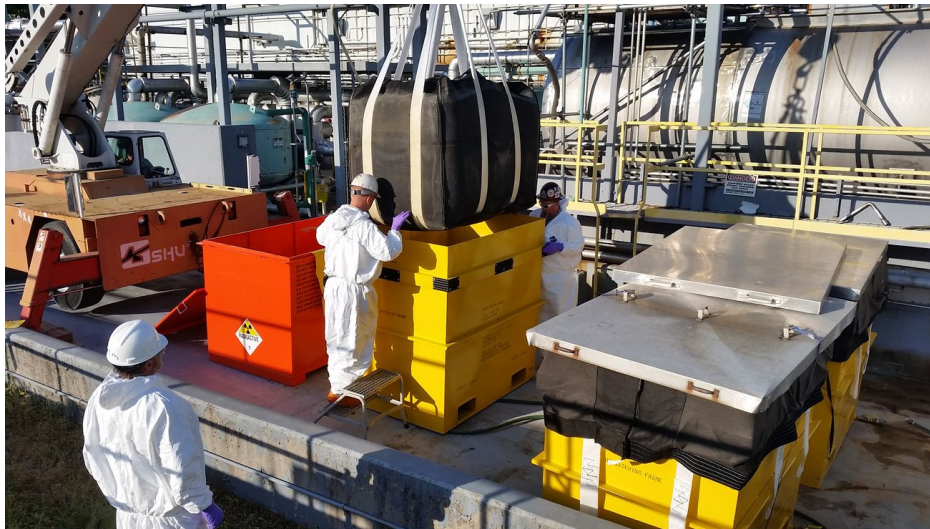
Geotextile water permeable package and frame system designed to dewater hazardous soils and contain solids to be sent for disposal.
